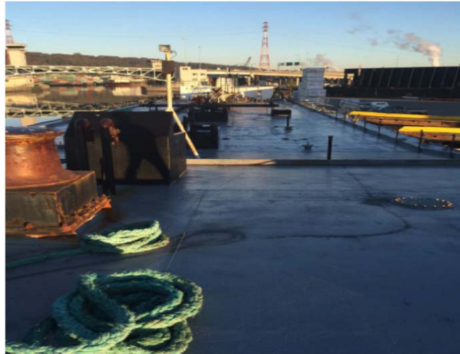
Tank Barge Kenny
